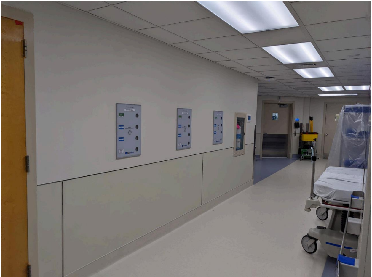
Exhibit 2.4 Interior view – Roger Williams Medical Center
