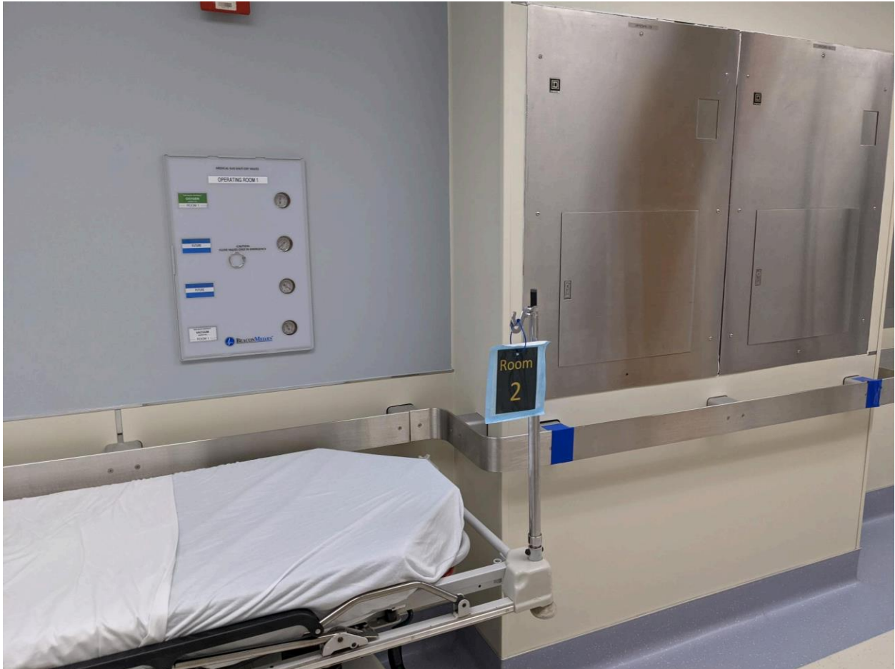
Exhibit 2.5 Interior view – Roger Williams Medical Center
